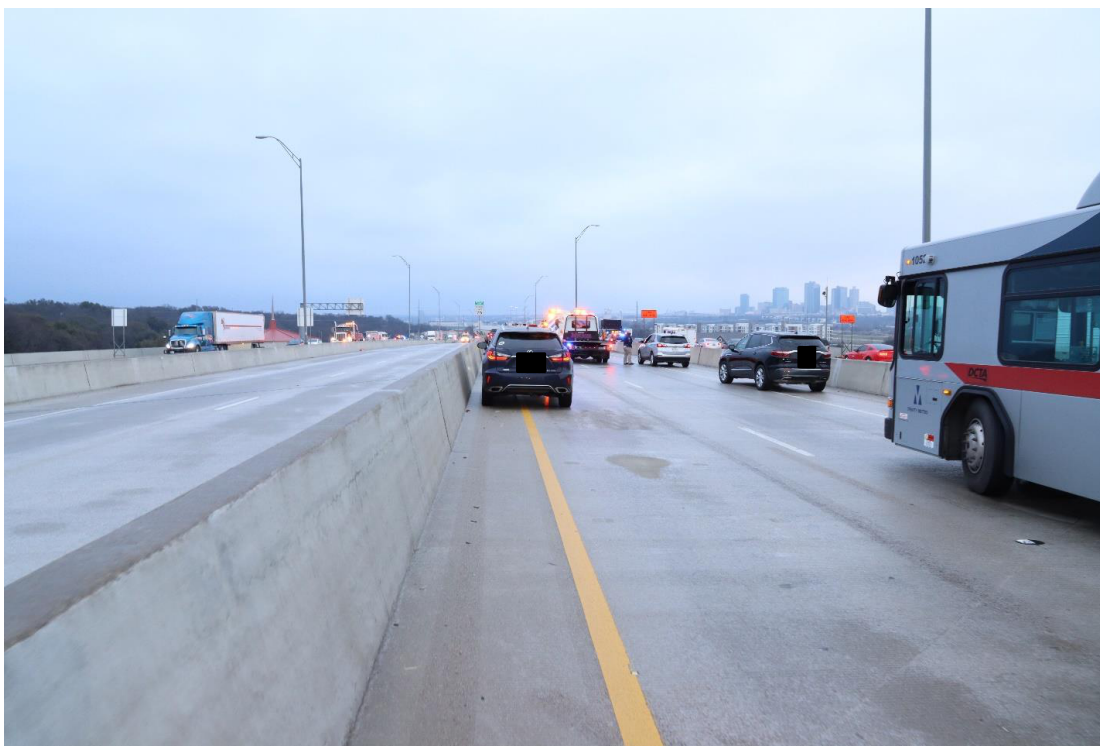
Highway Factors Photo 1 - View of I-35W southbound toll lanes standing on the left paved shoulder immediately north of the crash scene illustrating patches of ice on the roadway surface and top of the concrete barrier separating the I-35W southbound toll lanes and I-35W northbound toll lanes with the downtown Fort Worth skyline shown in the background looking to the south (Source: Fort Worth Police Department. Photo taken on February 11, 2021, at approximately 7:31 a.m.)
